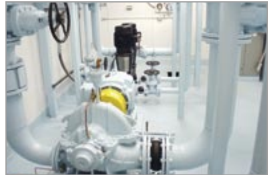
Above Ground Installation.
